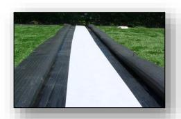
Apply a generous amount of BondMark adhesive to the seaming tape. Carefully, lay the two pieces of grass together so that the fibers or blades do not stick to the BondMark adhesive. Using NailMark, nail the stakes every 6" serpentine style along the seamed area. We recommend using BondMark adhesive when the temperature is 45° F or higher. You should plan to use approximately one tube of BondMark for every 15 – 20 linear feet of TapeMark seaming tape.
